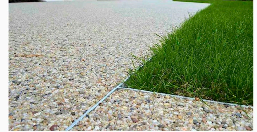
Resin bound gravel with stainless steel edge formers
